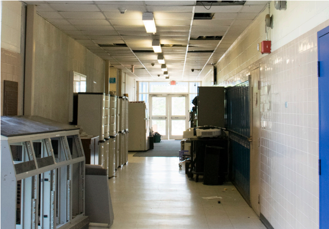
Old hallway lighting prior to the renovation.
